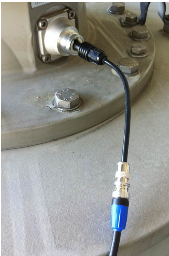
Connecting to a bushing tap using the adapter cable.
