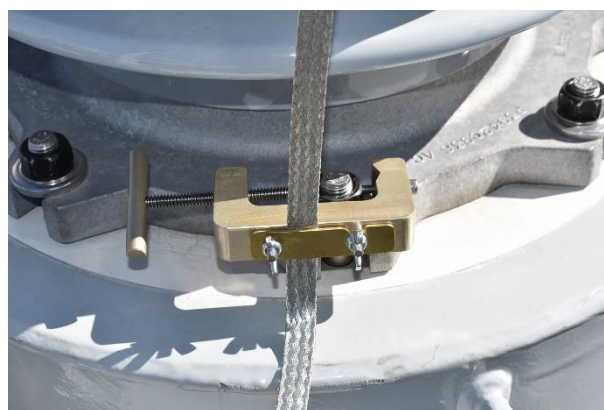
Earth connection to the ground clamp
